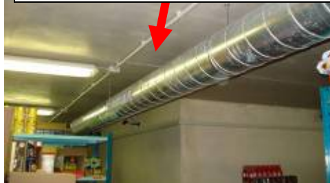
Shots show the type of ducting used clearly showing the jagged edges, which caused the cut Below is a shot of the work area.
